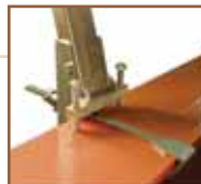
Stanchion installation complete
